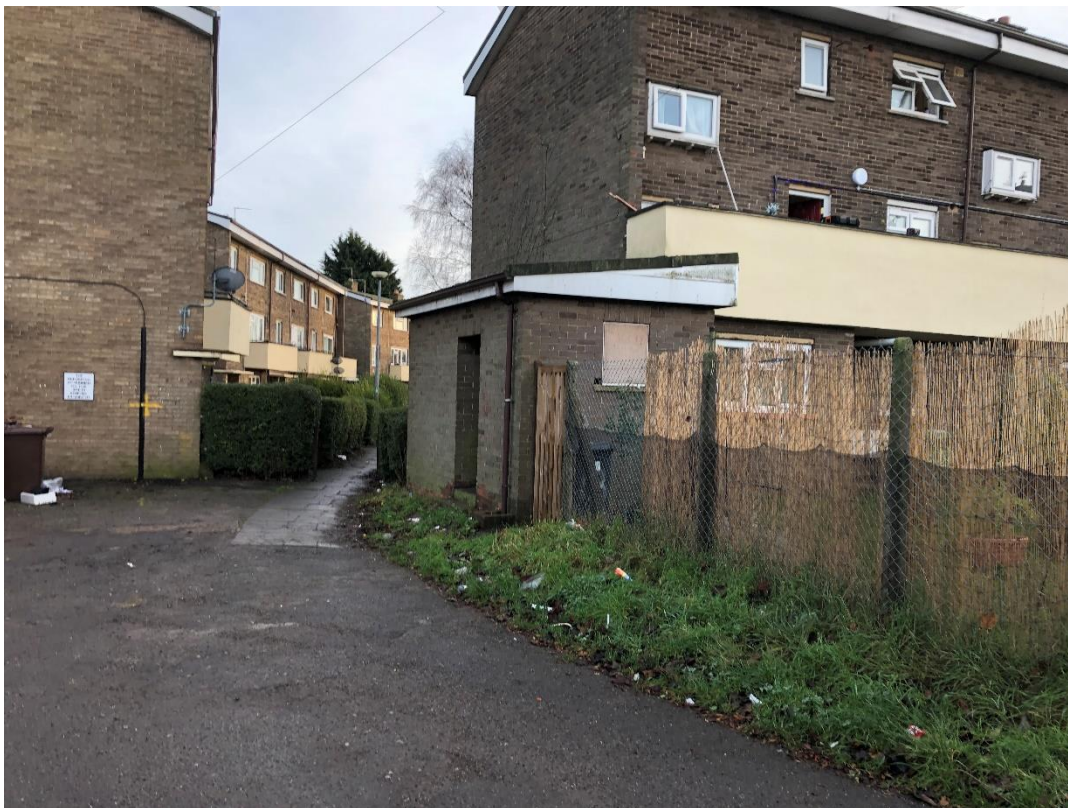
Bin store A and south west boundary of site with Windsor House
