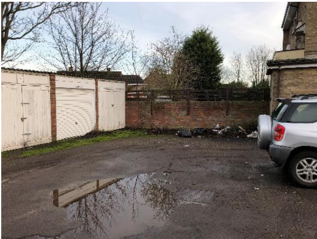
South east boundary wall with Stuart House to be replaced with fence
