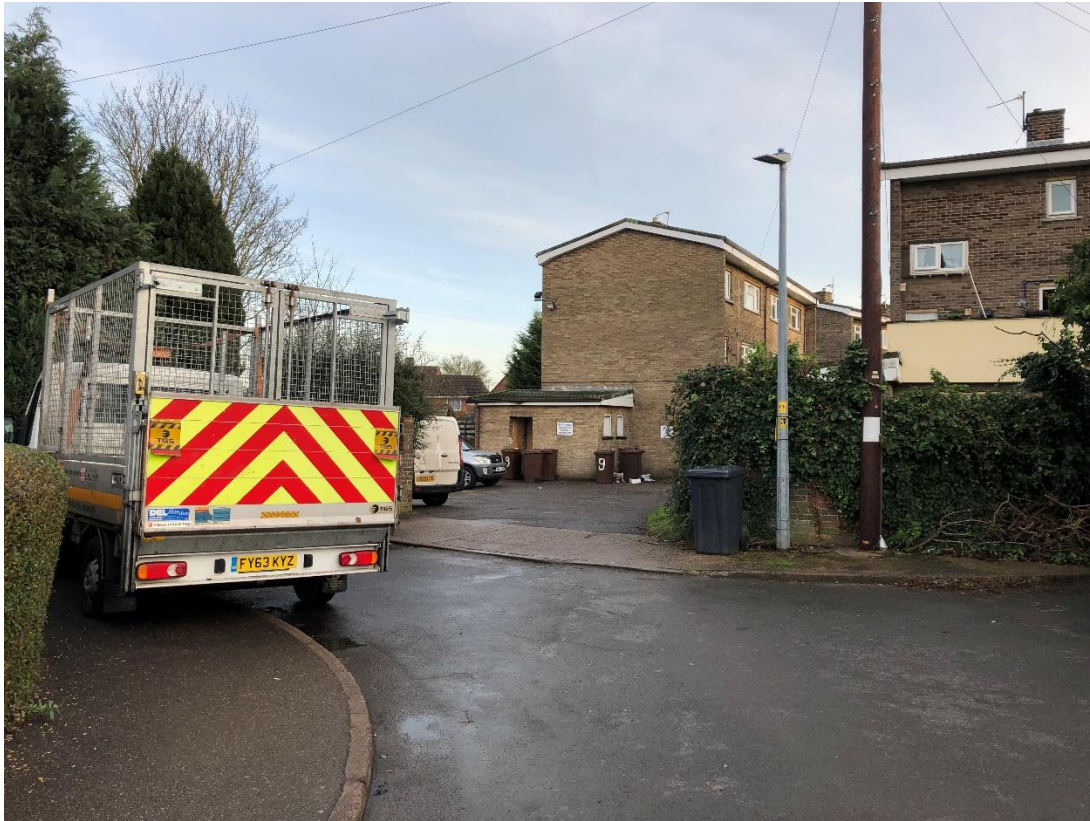
Site access, bin store B and side elevation of Stuart House
